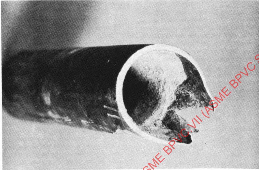
Figure 200.4.1-1 Scale Causing Overheating and Tube Failure
