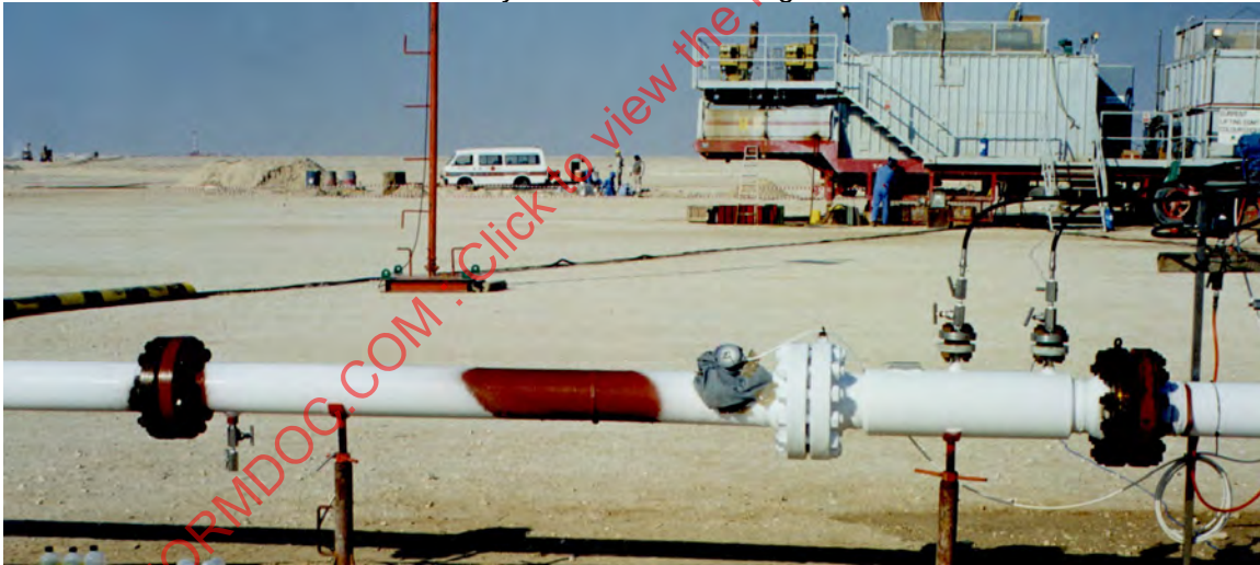
Fig. 9.1-11 PDO Wet Gas Venturi Meter With Frost and Frost Clear Sections Showing Thermodynamic Effects as Significant
