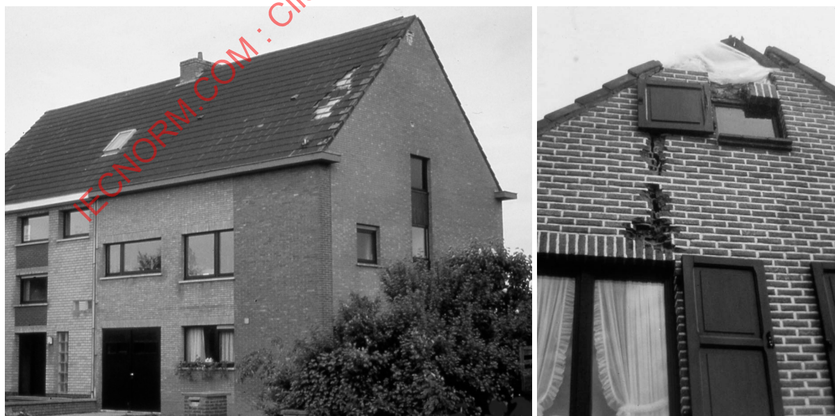
Figure 1 – Examples of roofs and facades damaged by lightning
