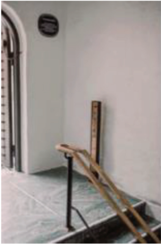
a) Raised platform and stairs
