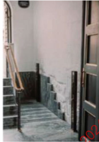
b) Lowered platform
