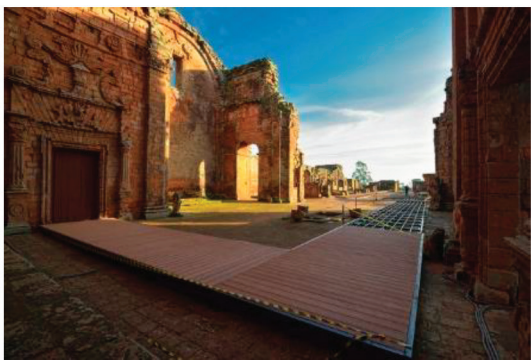
b) During the intervention works
