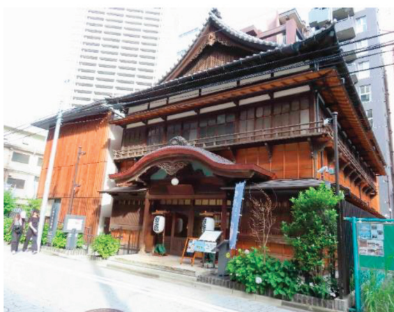
a) Stepped entrance to Kenban with ramped access to new annex on left
