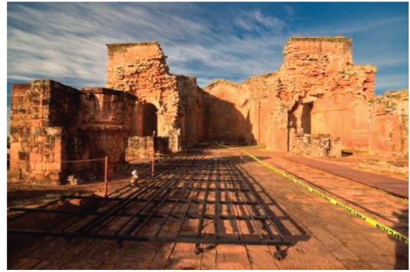
b) During the intervention works
