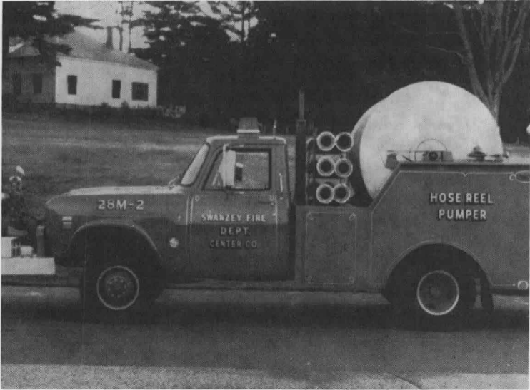
Figure B-1-9.1A. Apparatus with reel for large diameter hose. (Photo by Swanzezy, NH)
