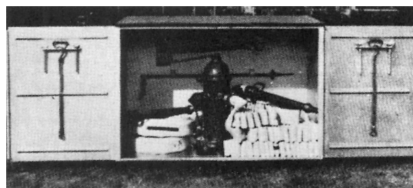
FIGURE A.4.3.5.3(a) Hose House of Compact Dimensions for Installation Over a Yard Hydrant. Construction can be Steel or Aluminum.
