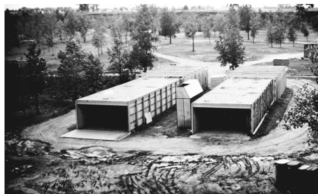
FIGURE 4.1.4(a) Overall view of 20 ft \times 100 ft (6.1 m \times 30.5 m) fire test building from exhaust end.
