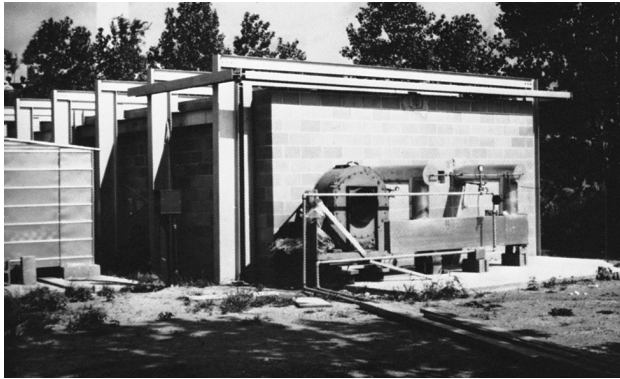
FIGURE 4.1.4(b) View of firing mechanism of fire test building.
