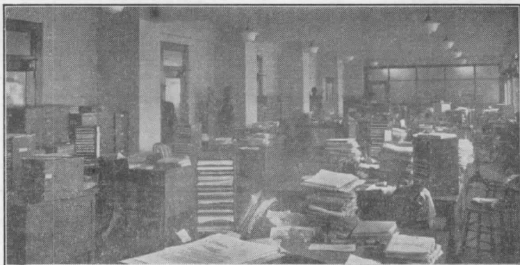
Fig. 1. Office with 6 lbs. per sq. ft. combustible contents. Cement finish floor, metal sash and frames, wood doors, wood furniture.
