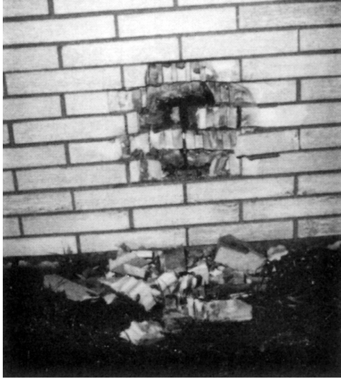
Figure 4-20.2 Damage to an outside brick wall caused by thermal expansion of an I-beam in the basement.
