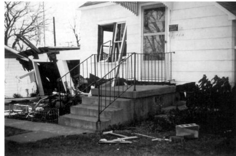
Figure 13-3.1 Low-order damage in a dwelling.
