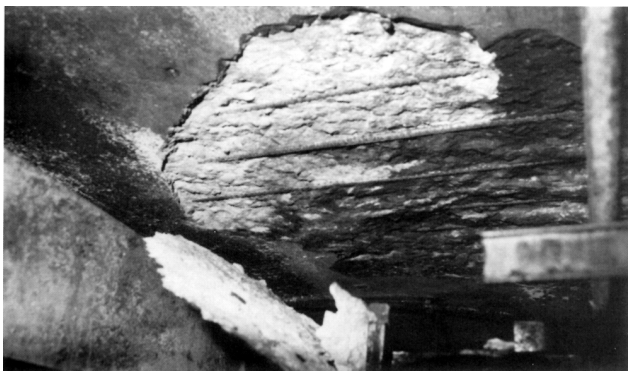
Figure 4-6 Spalling on ceiling.
