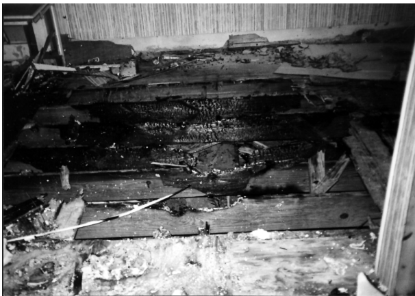
Figure 4-17.10 Saddle burn in a floor joist.
