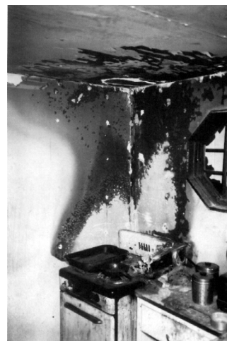
Figure 4-11 Clean burn on wall surface.
