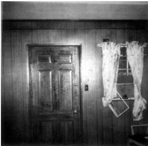
Figure 4-19.2 Blistering of varnish on door and slight scorching of draperies, the only indications of the natural gas flash fire.
